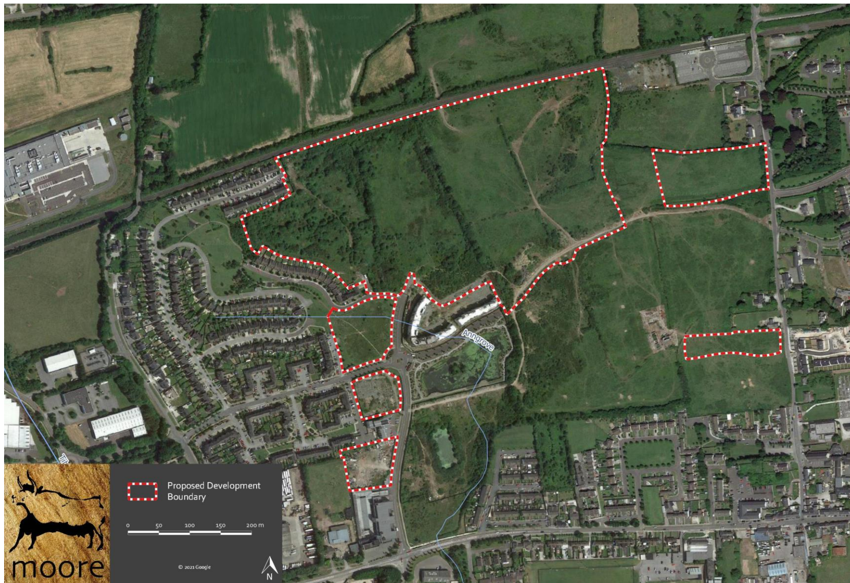
Figure 2. Showing the Project site on recent aerial photography, with the Woodstock (Anngrove) Stream visible to the south of the Project site.
